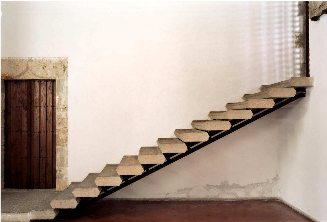
Fig. 5 Detail of the hexagonal steps of the Carini stone staircase
