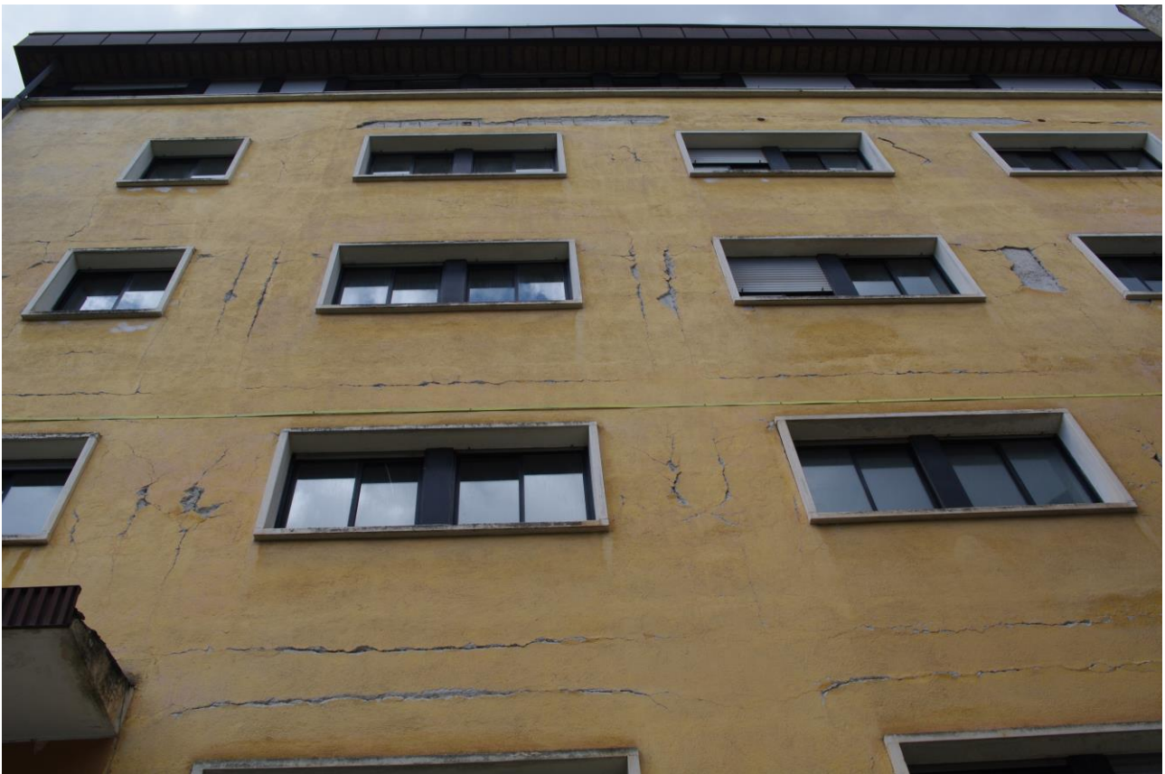
Fig.12 Back view of the building with earthquake damages
