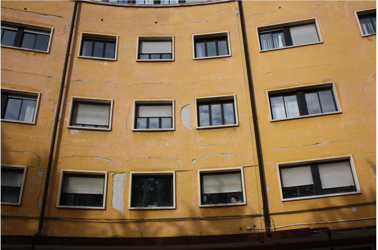
Fig.11 Front view of the building with earthquake damages
