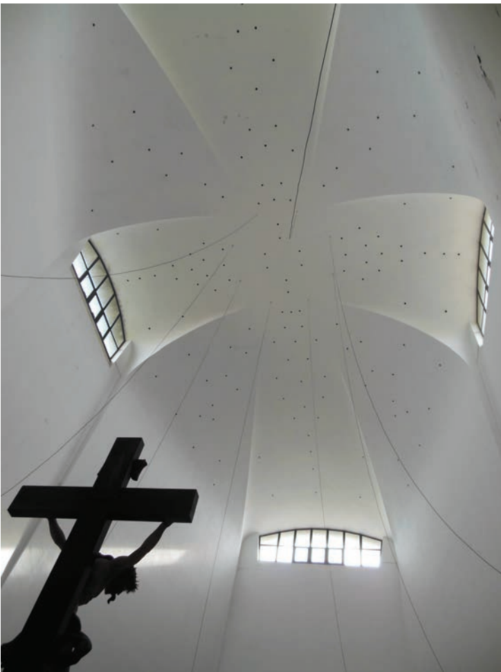
Fig. 5 The cross vault, aligned to main axes and joined to walls by large lunettes.
